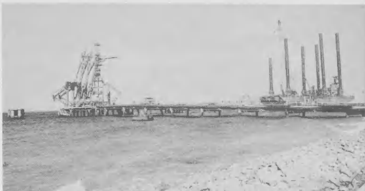
The Sea Berth built in 1969 is being upgraded to a more conventional pier to accommodate tankers of 250,000 dwt.
